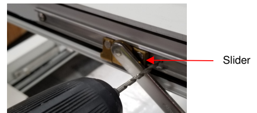
Figure 4: Roto Operator Drill Hole Location (Awning Shown)
