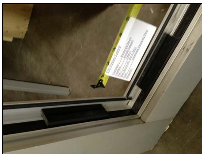
Fig. 3 – Setting block location in slab
