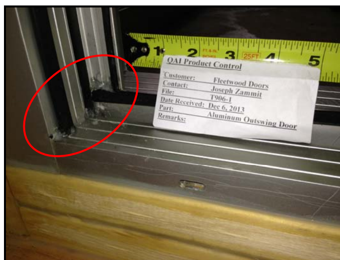
Fig. 17 – Silicone at weatherseals on sill
