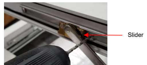
Figure 4: Roto Operator Drill Hole Location (Awning Shown)
