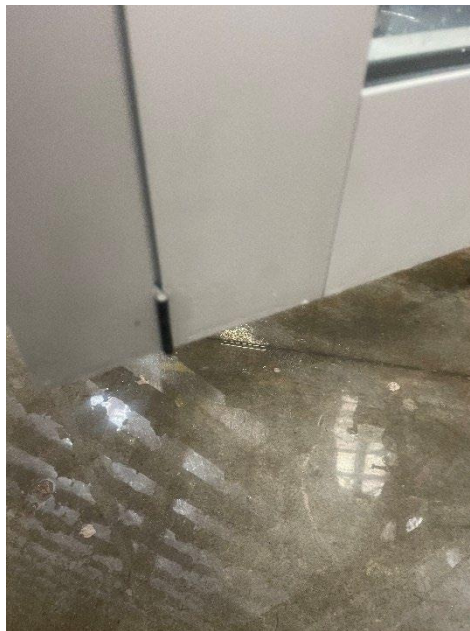
Photo No. 1 Added Sill Gasket Exterior Panel
