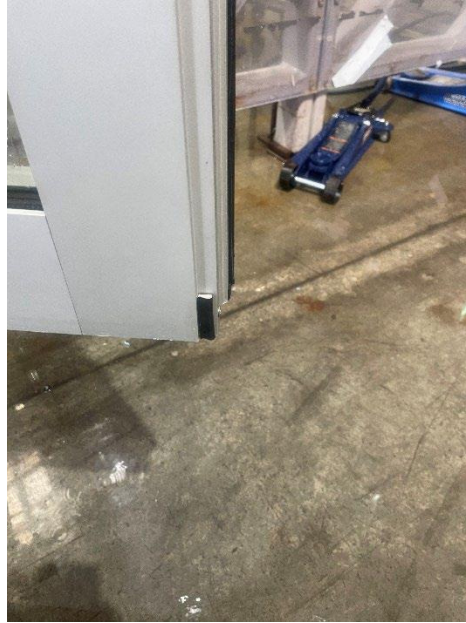
Photo No. 2 Added Sill Gasket interior Panel
