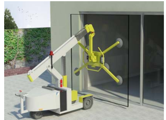
Figure 11: Glass Installation (after panel installation shown)
