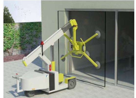
Figure 11: Glass Installation (after panel installation shown)
