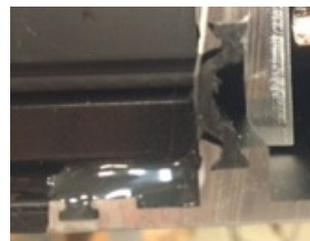
Figure 7: Seal joint thoroughly
