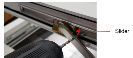
Figure 4: Roto Operator Drill Hole Location (Awning Shown)
