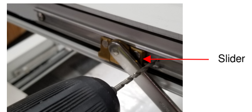
Figure 4: Roto Operator Drill Hole Location (Awning Shown)
