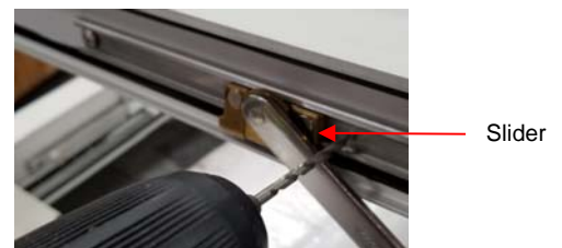
Figure 4: Roto Operator Drill Hole Location (Awning Shown)
